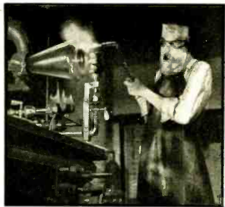
Fig. C. A blowtorch helps fuse screen to slowly-revolving television-tube envelope; while gas flames from all sides maintain glass at even heat. It is this operation which the cover painting depicts in colors.
